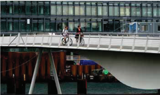
Above: Cycle and foot bridge, Copenhagen, Denmark
