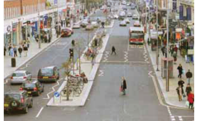
Above: High Street Kensington, London. De-cluttering, removal of obstacles to pedestrian movement, cycle parking provision among other measures. Recorded accidents considerably reduced following implementation.
